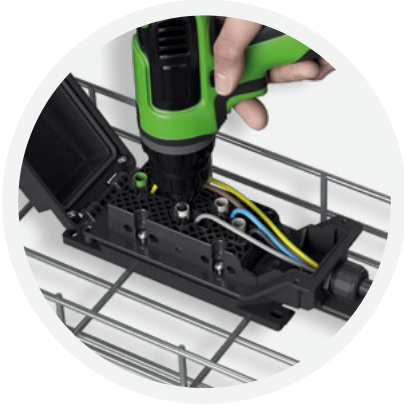
Copper displacement connection of the cable
